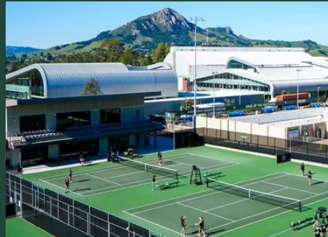
Comerford Pavilion Completed November 2024
