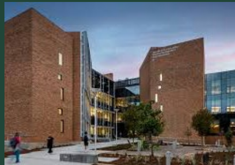
Robert E. Kennedy Library Completed September 2025
